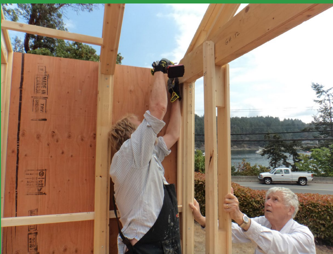
Gable header (GH) placement and installation.
