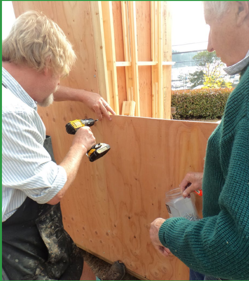
Attaching 8 foot panel between door and window openings.
