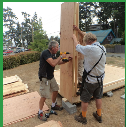
Attaching corner start to panel.
