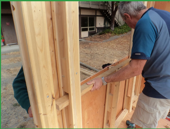
Adjusting bottom plate on window opening.
