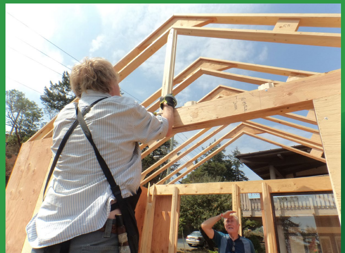
Adding structural support to the rafter and providing a bedding for the walls to be fastened.
