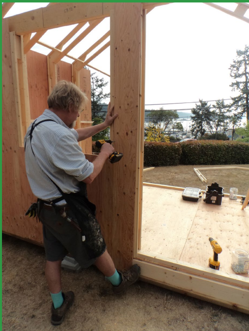
Attaching 8 foot panel between door and window openings.
