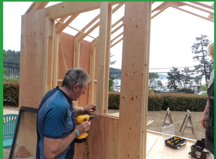
Preparing the opening for the placement of the window.
