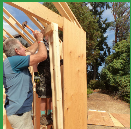
Gable header (GH) placement and installation.
