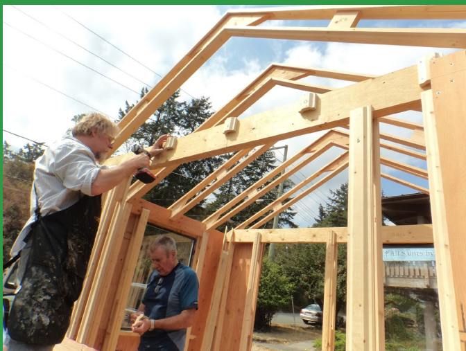
Adding structural support to the rafter and providing a bedding for the walls to be fastened.
