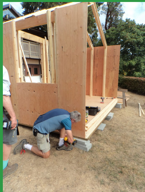
Completing fastening of the wall panel beside a 4' x 4' window opening.
