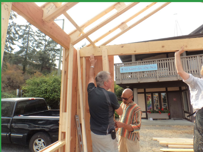
Installing gable end header.
