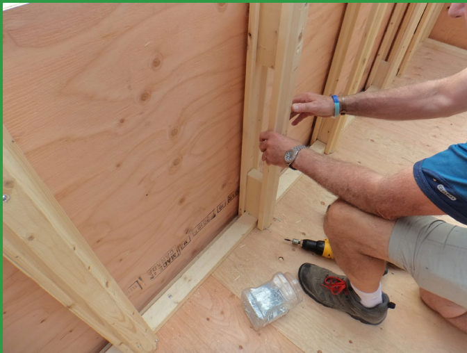
Adding structural support to the rafter and providing a bedding for the walls to be fastened.
