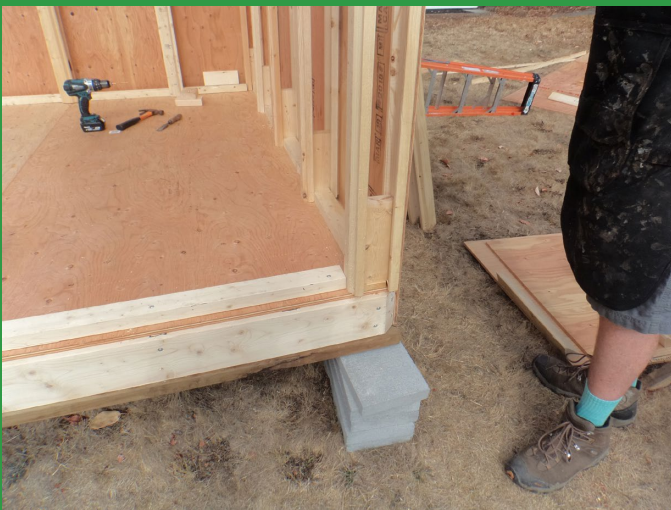
Attaching plywood to spacers block to stud.
