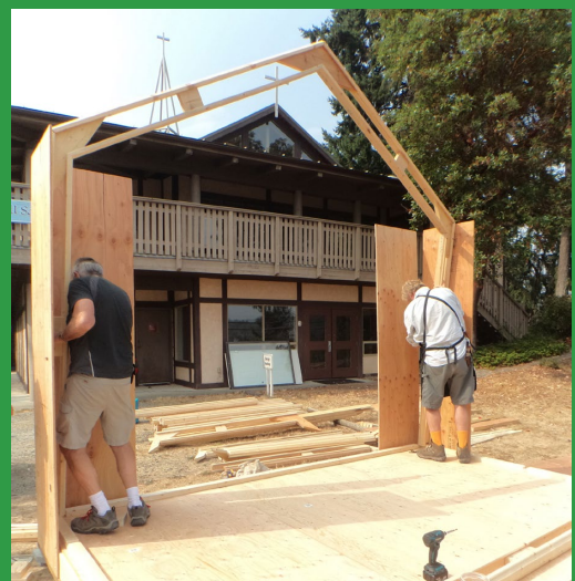
Assembling first arch with corner plywood for bracing.
