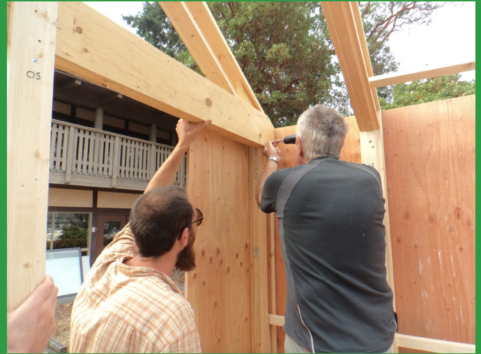
Installing first gable end start to bottom plates.
