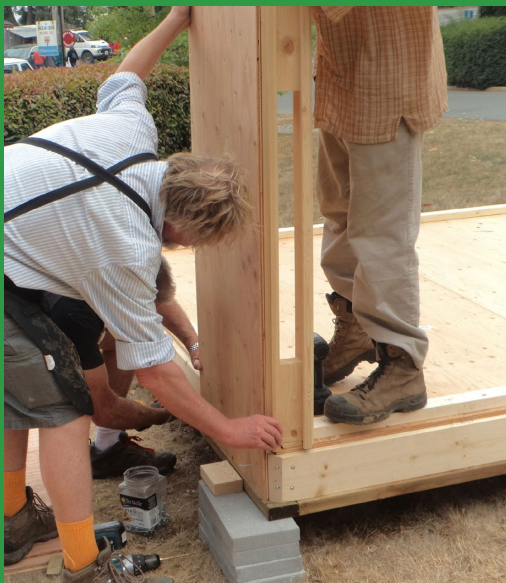
Just checking position of first arch on platform.
