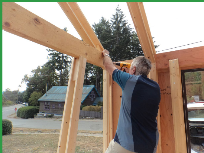
Gable header (GH) placement and installation.
