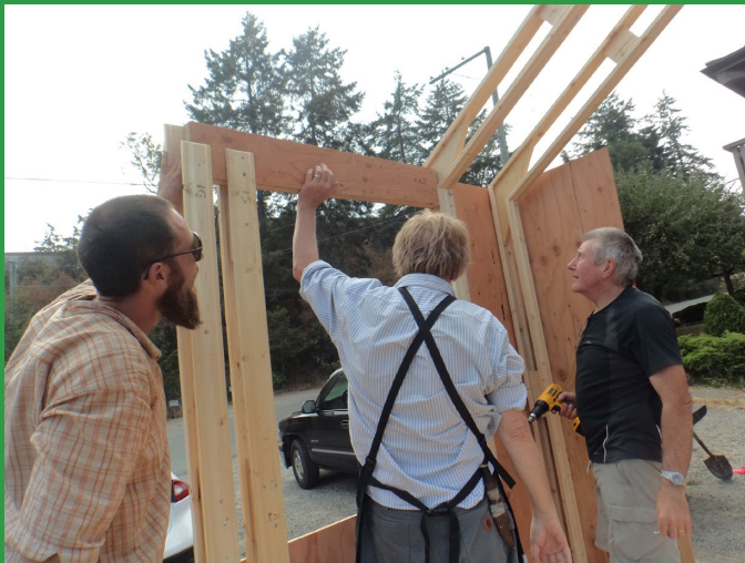
First step installing window header in the 8 foot wall.
