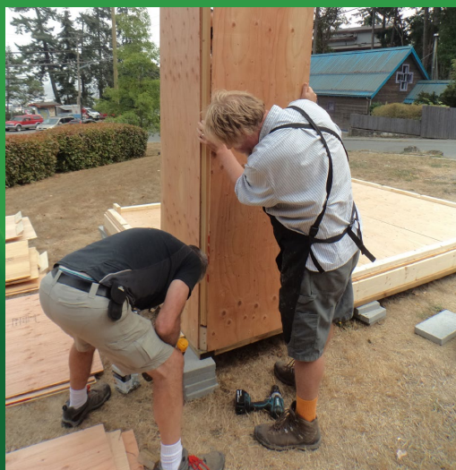
Checking corner position.
