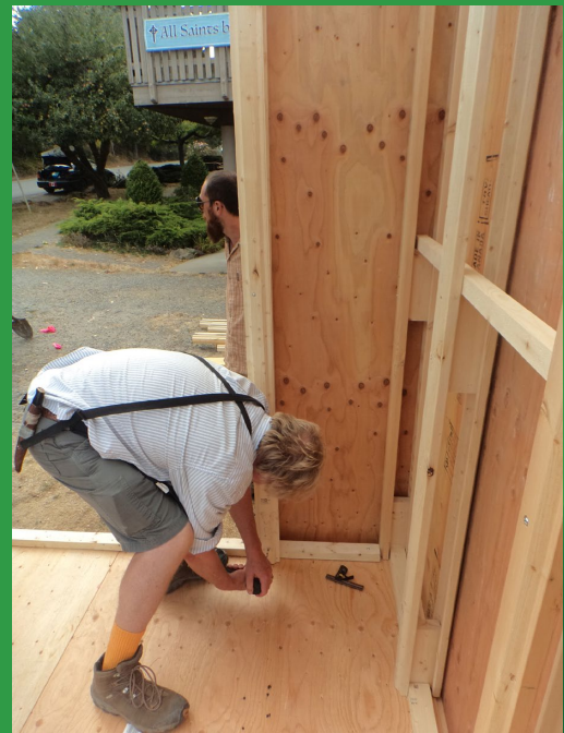
Installing first gable end start to bottom plates.
