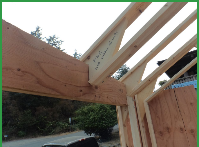
Gusset WG on rafter has been changed to gusset WWG.
