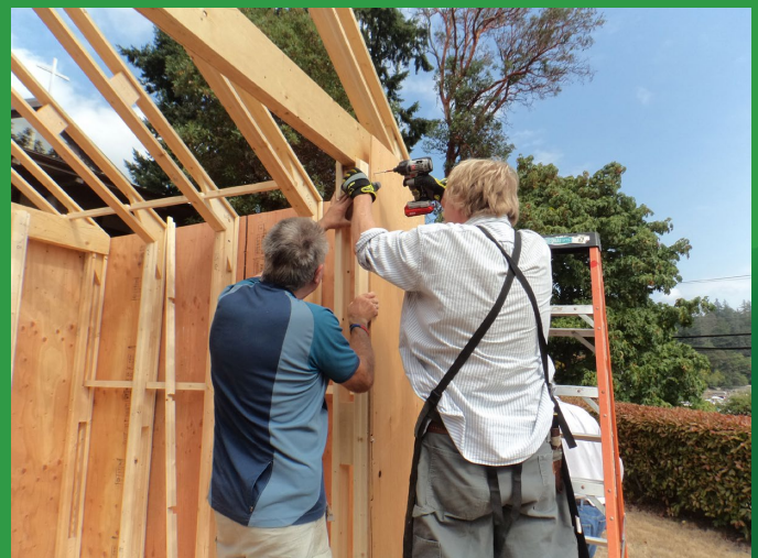
Gable header (GH) placement and installation.
