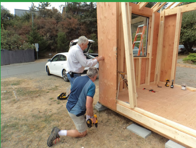
Gable header (GH) placement and installation.
