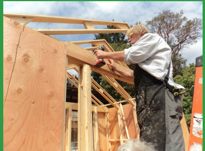
Adding structural support to the rafter and providing a bedding for the walls to be fastened.
