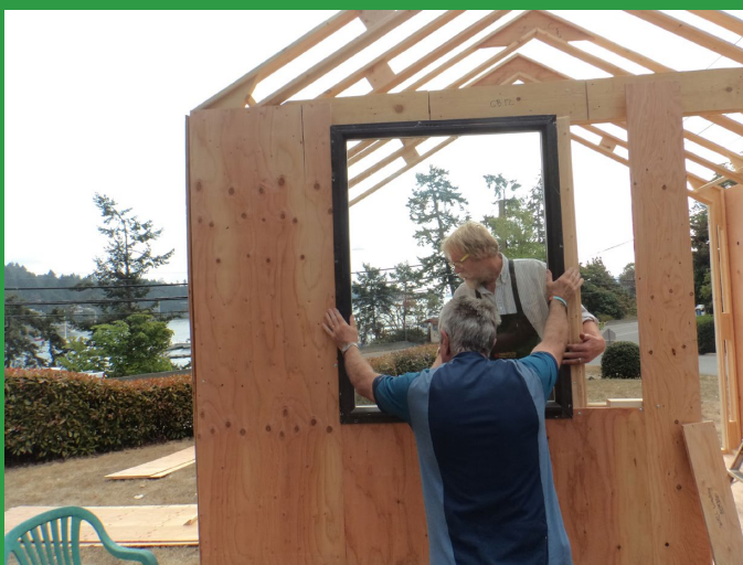
Gable header (GH) placement and installation.
