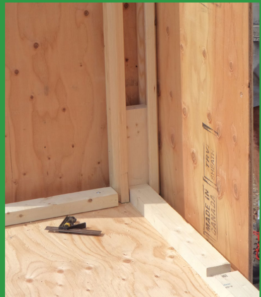
Corner positioning of start and bottom plates.
