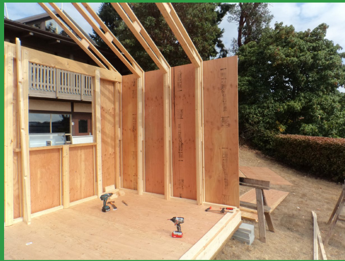
Completing fastening of the wall panel beside a 4' x 4' window opening.
