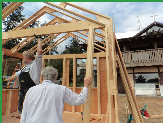
Gable header (GH) placement and installation.
